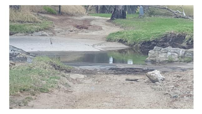
3.20 Given the high velocities, a volume of silt and debris material estimated well over 1000 tonnes has been deposited in various sections of Dry Creek. The photo below shows the inundation by material of Council's Gross Pollution Trap, but also shows the sheer tonnes of material now relocated from upstream into the lower dry creek catchment.
