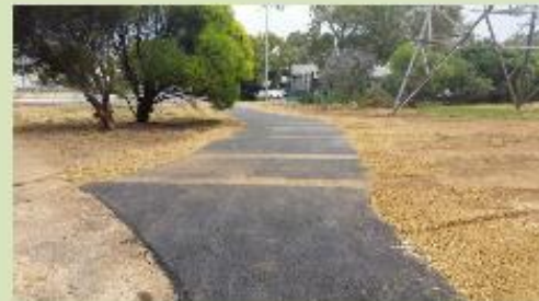
Gawler Street, Salisbury, New Footpath
