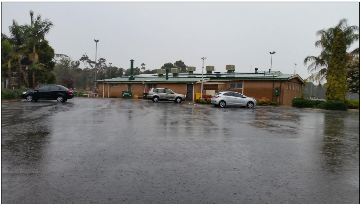
Photo 4: Salisbury Bowling Club Building to be retained
