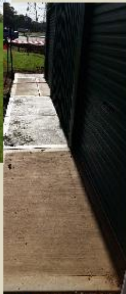
After – New concrete
