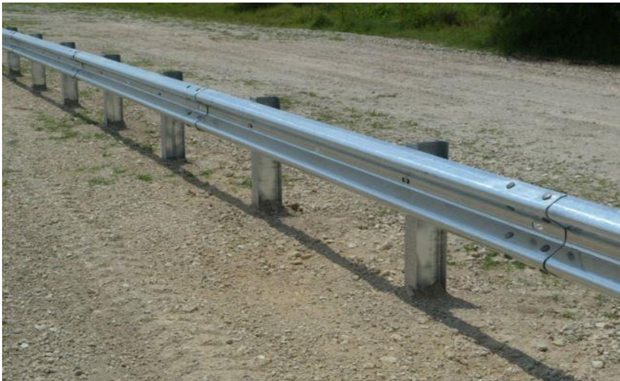
AN EXAMPLE OF STANDARD W-BEAM GUARD-RAILING TO BE INSTALLED FOR PERIMETER PROTECTION FOR THE OUTDOOR PLAY-AREA OF A CHILDRENS CRECHE
