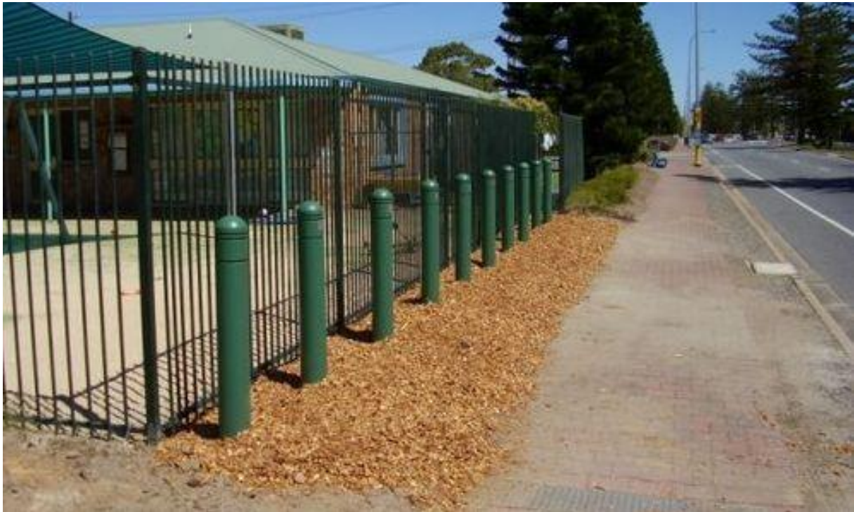
AN EXAMPLE OF THE INSTALLATION OF THE OMNI STOP BOLLARDS FOR PERIMETER PROTECTION FOR THE OUTDOOR PLAY-AREA OF A CHILDRENS CRECHE
