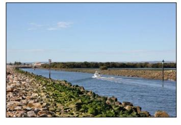
There is a northern and southern breakwater forming the channel. The southern breakwater is in poor condition due to tidal/storm activities and from bow wash from vessels entering and exiting the channel. It must be accessed from the water making repairs challenging and costly. Recent works have been undertaken to repair and renew the northern breakwater – which is accessible via land.
