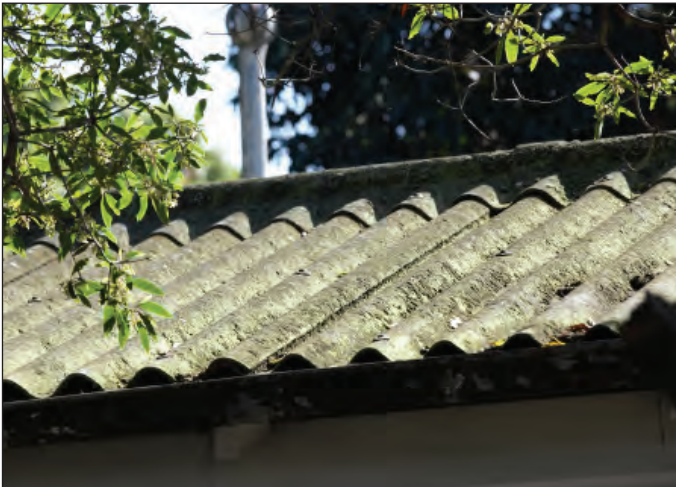
Corrugate asbestos cement roof cladding
