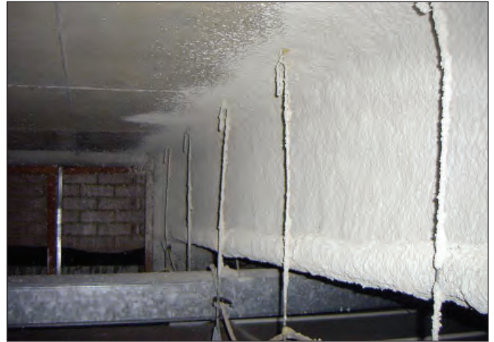
Sprayed asbestos
