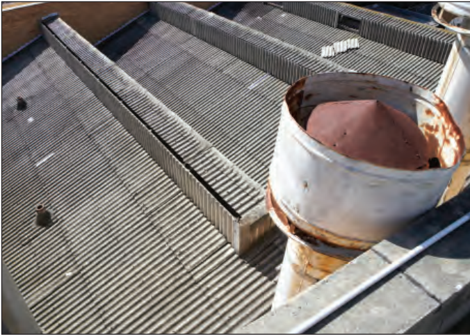
Roof with corrugated asbestos cement roof cladding.
