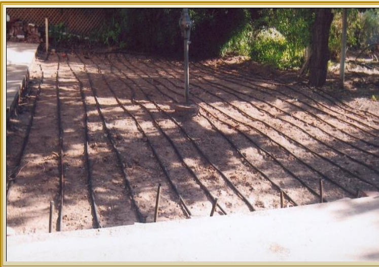
Soaker hose at 20cm depth, prior to top-dressing
