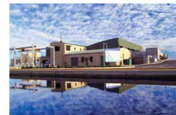
Bolivar Treatment Plant
