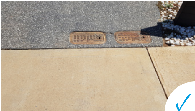
Services in driveway pits between the footpath and the property boundary where existing footpath is being retained.
