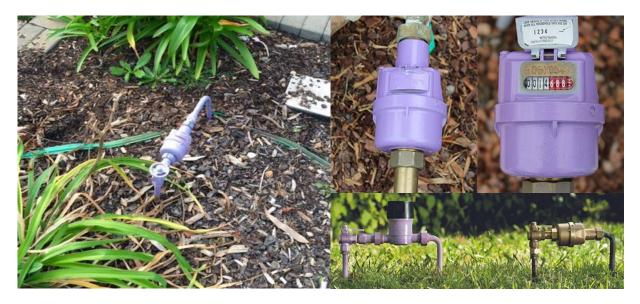
On the face of the meter you will see a series of numbers. The numbers measure the amount of water used in kilolitres and litres. The black numbers measure kilolitres (thousands of litres) and the red numbers measure litres. When providing your Salisbury Water meter reading please provide all numbers to us.
