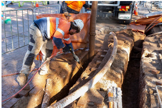
Trenching works being undertaken to install underground infrastructure to accommodate new LED lighting, CCTV, Wi-Fi and irrigation
