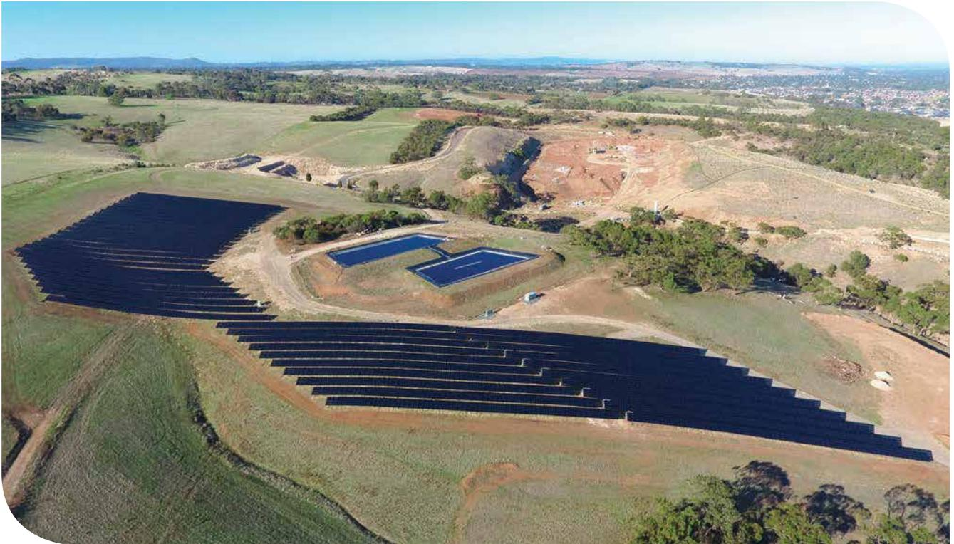
**NAWMA's Uleybury Balefill and Renewable Energy Park is the first combined solar - landfill gas farm of its type in Australia and continues to generate power for the local community using over 11,000 solar panels and gas extracted from 18 vertical wells, and a network of horizontal wells in the active cell area.**
