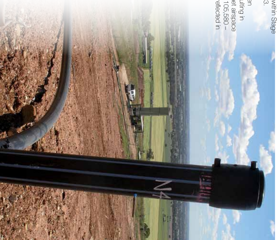
A landfill gas extraction well connected to a gas flaring system
